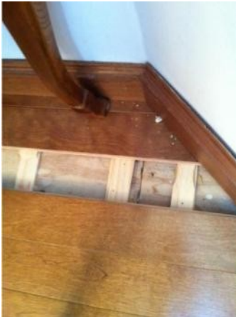
Don't use paint sticks to shim a bad subfloor
